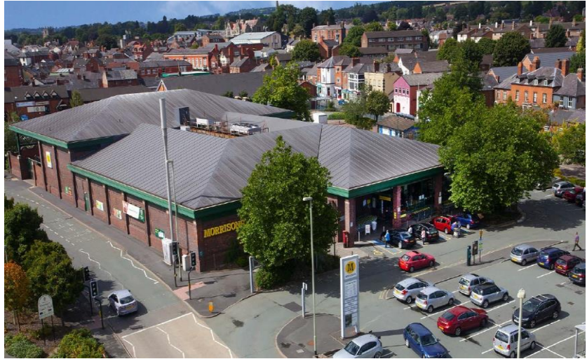
(Prior to supermarket closure)
