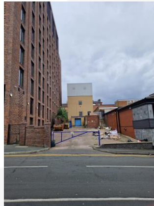
Rear elevation, with adjacent student accommodation
